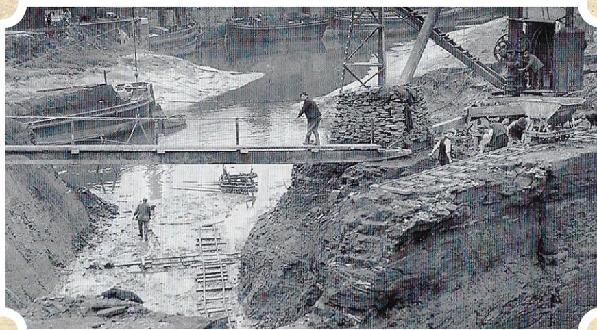
In 1912, the decision was made to cut through the neck of the lan where the River Dibbin entered Bromborough Pool. This gave easier access for vessels entering Port Sunlight Dock without having to pass barges moored at the wharf. This picture, taken from the New Chester Road, shows the mammoth task of cutting through the sandstone bedrock to form the new channel
