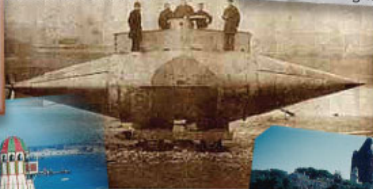
Old Merseyside Submarine The original Resurgam, designed by the Rev G Garrett in 1878, sank in 1880 found by fishermens net in 1995.
