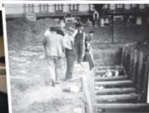
Building Air Raid Shelters & Tank Traps in Wallasey 1936
