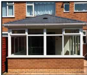
After Lightweight Roofing
