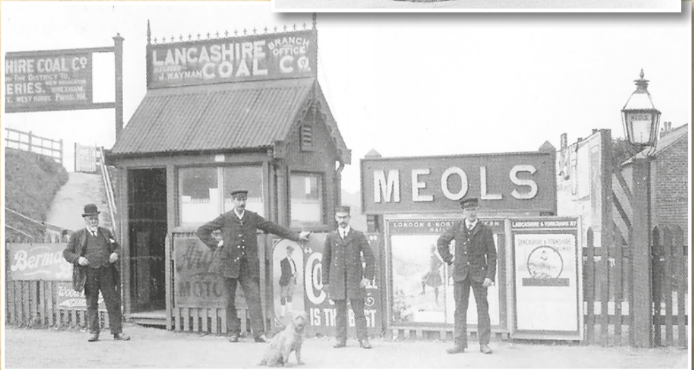
Above: 1919. The Station Master; staff and dog pose for a photograph on the platform of Meols Station. The slope on the left led up to Birkenhead Road.
