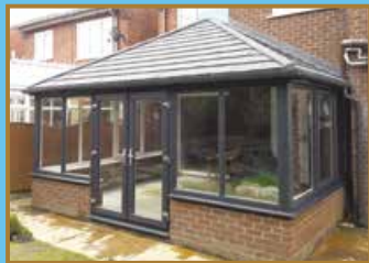
AFTER ROOF INSTALLED
