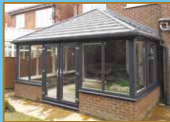
AFTER ROOF INSTALLED
