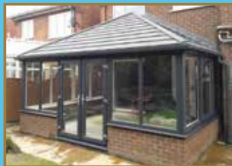
AFTER ROOF INSTALLED
