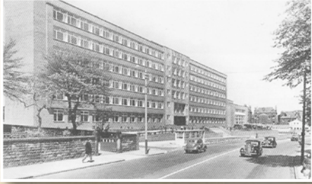
Above. Birkenhead Technical College in Borough Road Birkenhead started construction on 29 September 1949 and the foundation stone was laid by Queen Elizabeth on 3 May 1950. Work cost £653,000 and was completed in 3 years. Top photograph shows the shell and the bottom one completed in 1955.
