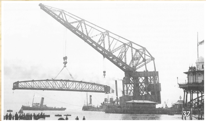
Right. 1920 a crowd has gathered to watch the giant crane "Mammoth" lift the 150 ton gangway for New Brighton Pier on 2 December 1920. The gangway was to connect the floating stage with the pier which is seen on the right.
